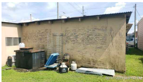
Rear Detached Shed
