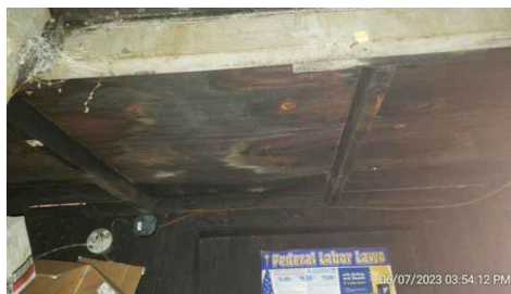
Rear Detached Shed
