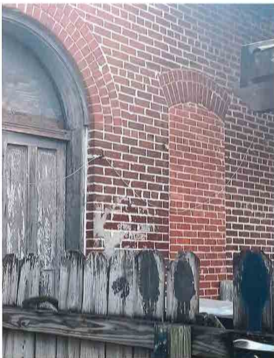
Back of Building 225 Fowlkes Example of Masonry Infill
